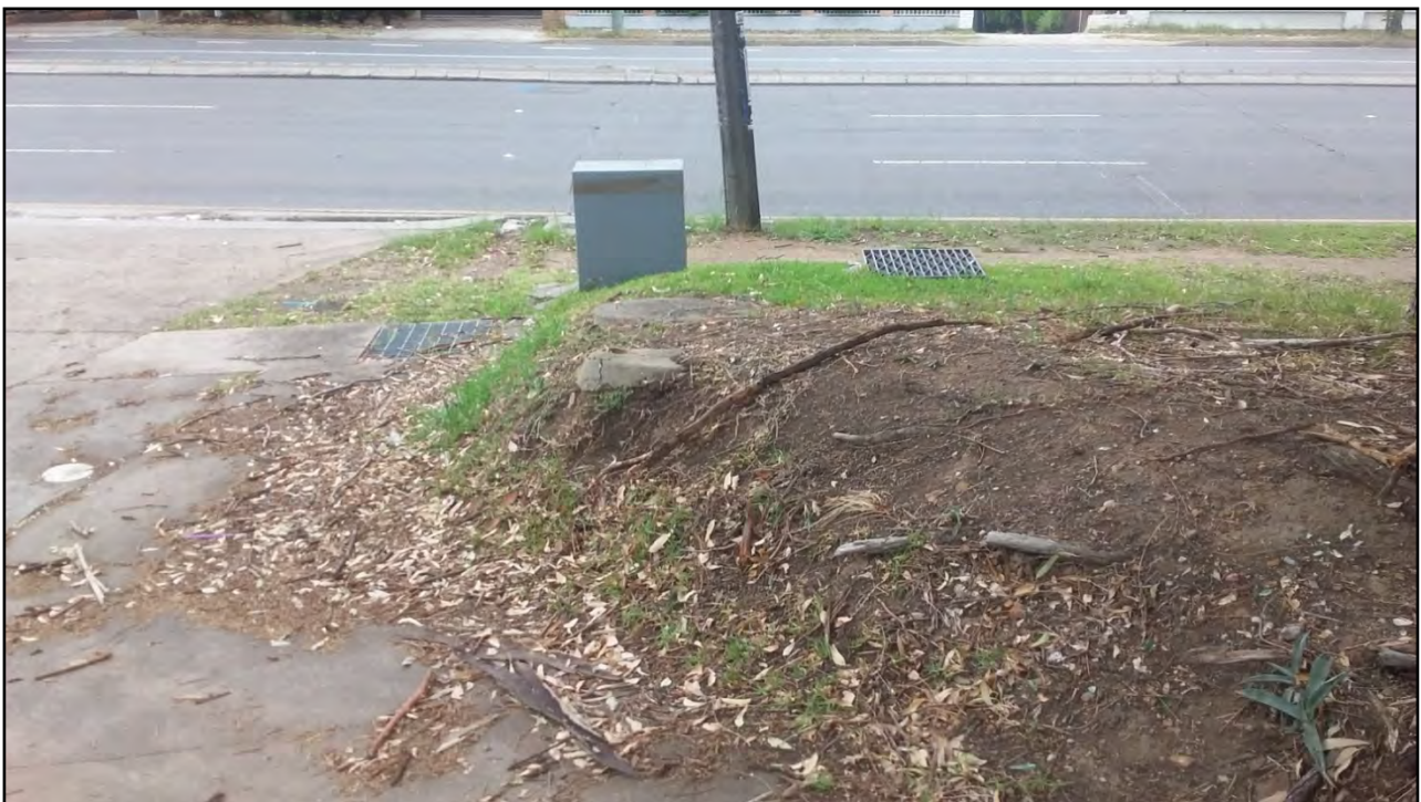
Photograph 8 – Site drainage at southern exterior of the Site, as observed on 19.12.2017
